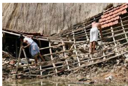
Destruction post Aila
